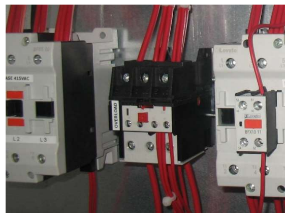
Thermal overload protection ALL models
