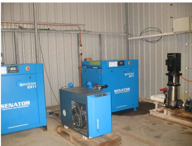
2 x 11KW, 1 x 7.5KW pump compressors powered by POLYPHAZ
