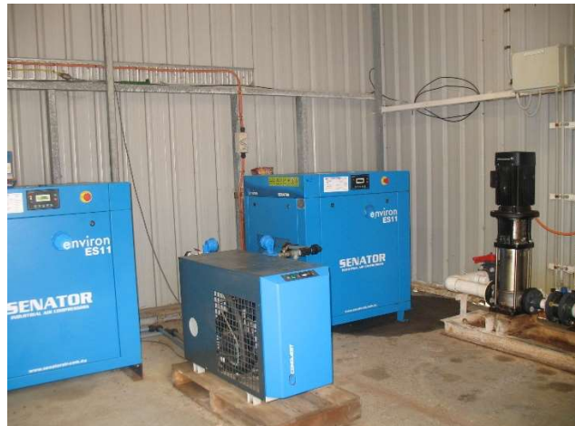
2 x 11KW, 1 x7.5KW pump compressors powered by POLYPHAZ
