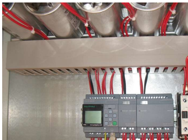
High spec power capacitors standard with R & HR converters
